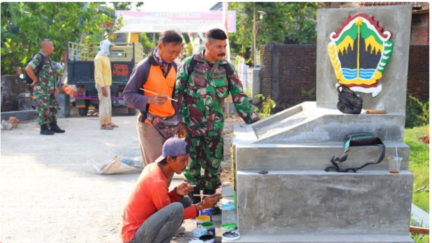
(Foto istimewa ) pengecatan tugu prasasti tmmd reg 116
